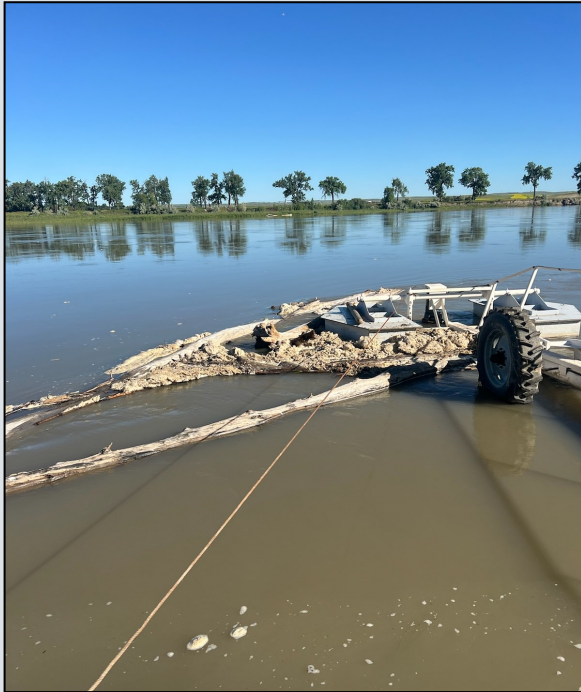
Large debris often built up on pump sites located downstream of the Fort Peck Dam during the second high peak in June. Picture provided by Dana Berwick.
