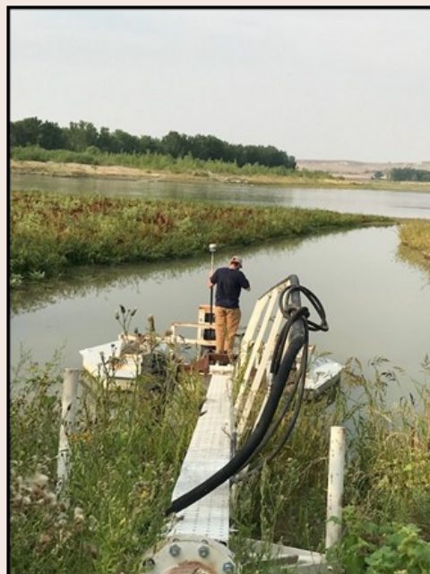
A side channel intake pump site. The intake will be laden with silt after an extreme high flow event. The silt will be difficult and dangerous to remove during the immediately following low flow.
