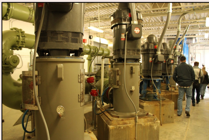
Intake pumps in the Missouri River supply the Assiniboine Sioux Rural Water Supply System with water. This System serves the Reservation and much of Northeastern Montana with necessary domestic, municipal, and stock water.
